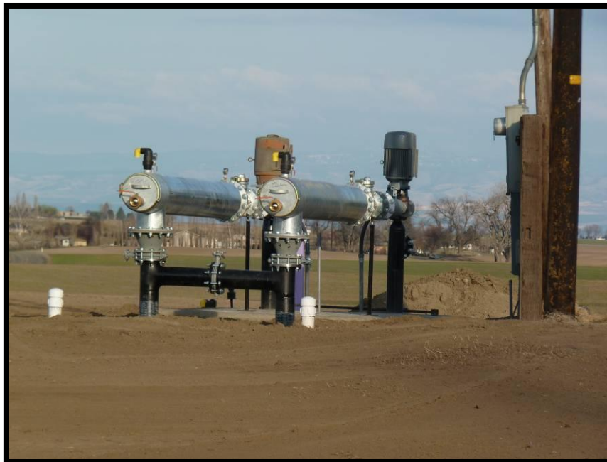
A new pumping station complete with concrete pad and new power service panel
