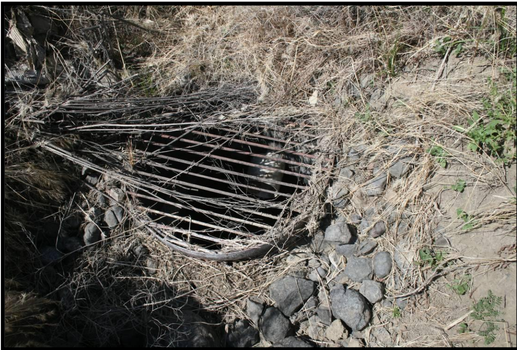
Maintenance of deteriorating grade control and intake structures are also part of the annual maintenance costs for GFID#13
