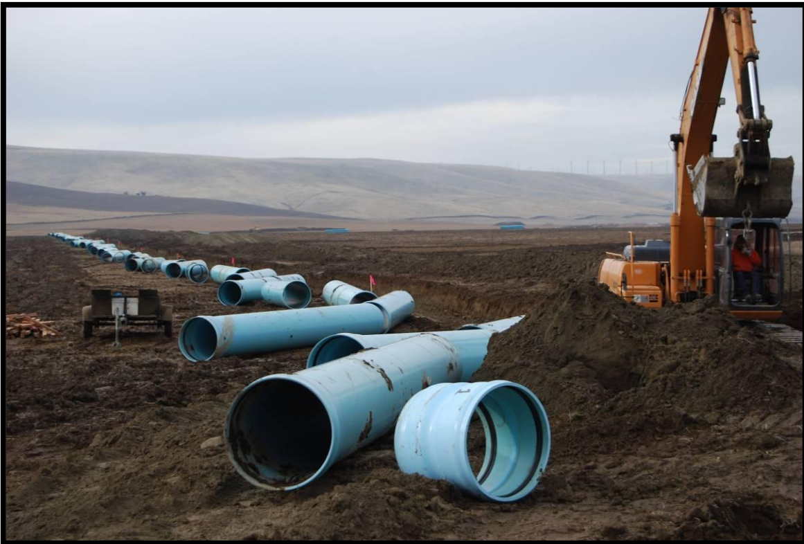
Pipe staged for installation as excavator operator prepares the trench
