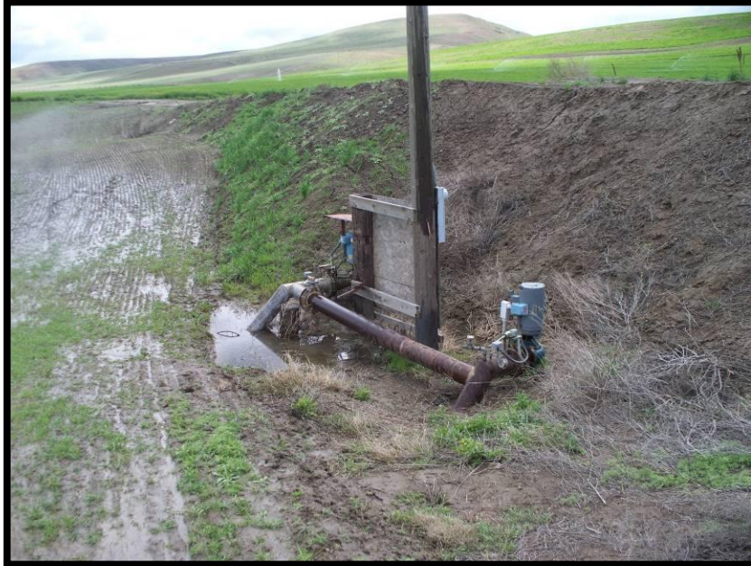
Example of a pumping station prior to modification
